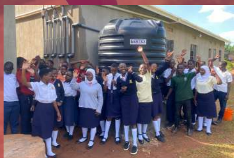
Rainwater Filter System
